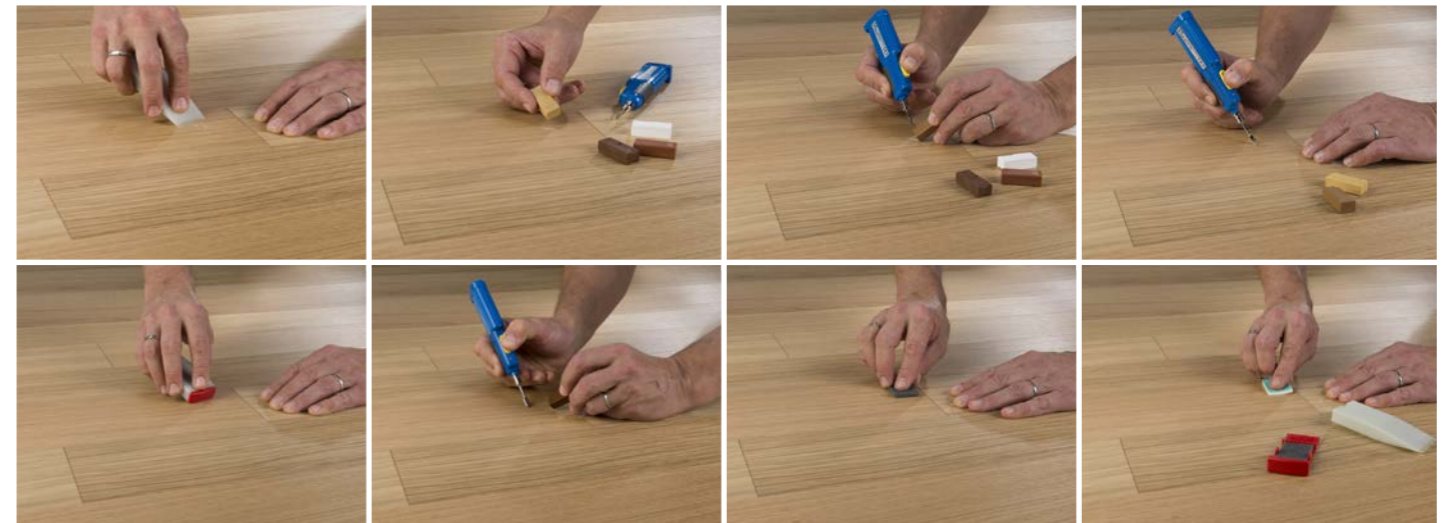
The process for repairing the floor with a melt gun with wax
